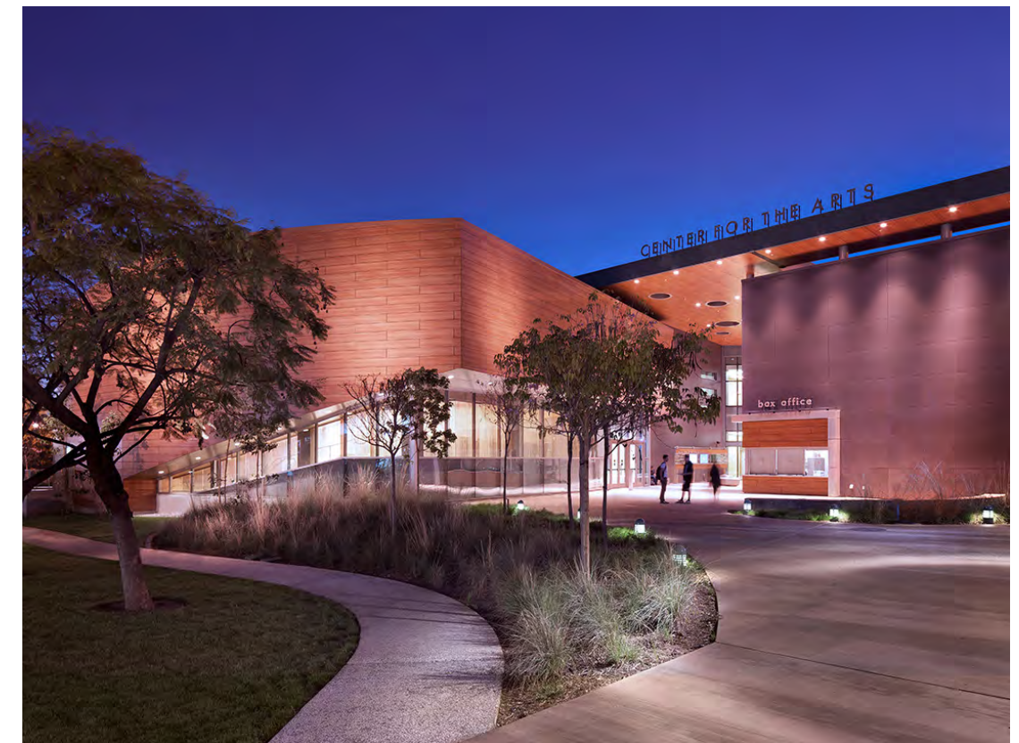
The LEED-recognized Center for the Arts building
